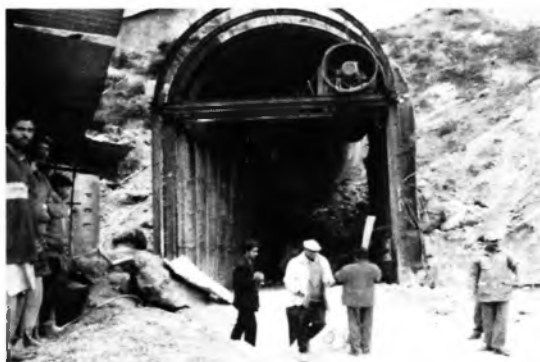
Collapsed at Portal 2 of Tunnel No. 1
